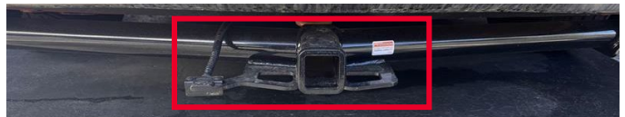
TOW HITCH HARNESS INSTALLED
