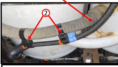
Retain the Return Fuel Line to the pressure relief valve hose using two Dual Clamp Zip Ties as pictured. **Maintain a minimum of 2" of clearance between the fuel line and clamp used on the pressure relief valve hose**. The red tape on the Return Fuel Line indicates the proper retention locations.
