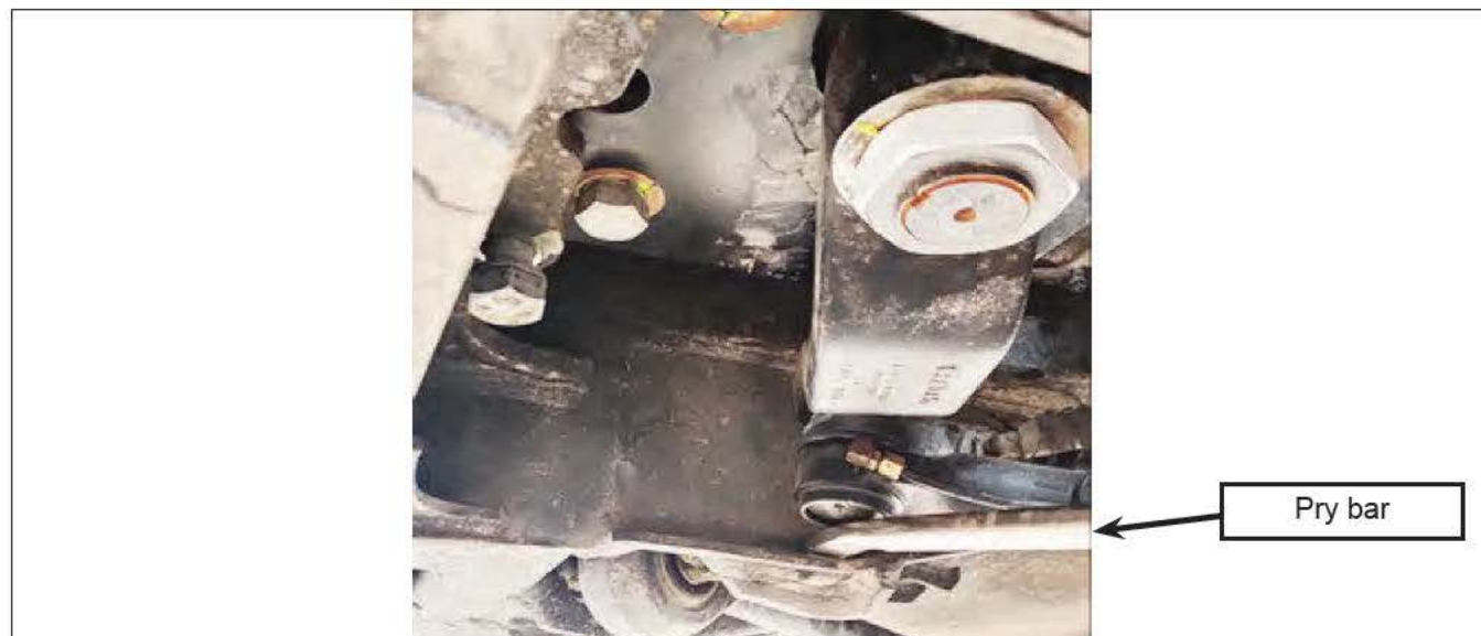
Figure 5 - Use a Pry Bar to Lift Slightly the Gear Box Mounting Plate
