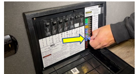
Remove Awning Fuse From Fuse Panel
