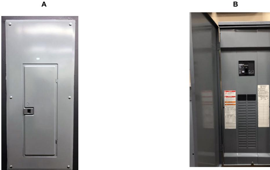
3. Using a properly rated voltage sensing device, verify the absence of voltage.
