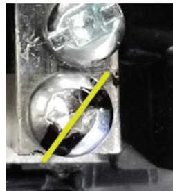
If the PoN connector **DOES MOVE**, the clamping screw in the PoN connector must be tightened.
