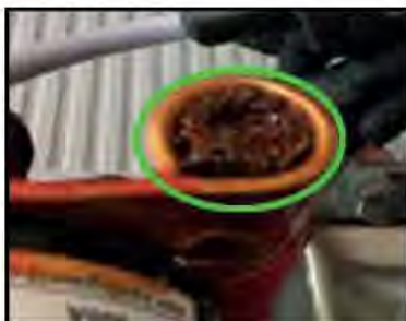
Figure 9 - Conform Application of N67314 NCP-2 Anticorrosive Compound
