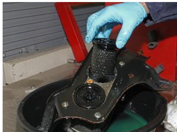
Figure 54 – Remove Old Filter Covers and Elements
