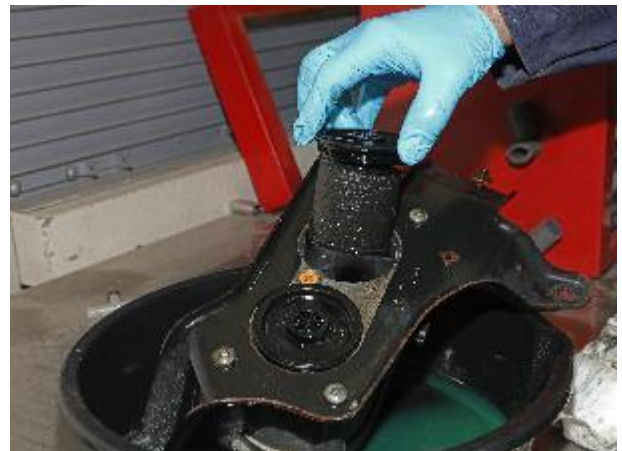
Figure 54 – Remove Old Filter Covers and Elements
