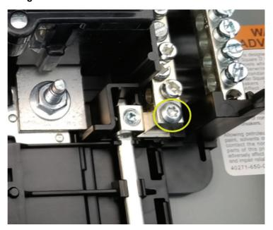
Use the screwdriver to turn the right neutral bar screw alternating clockwise and counterclockwise, while inspecting for movement on the PoN connector. See Figure 14.
