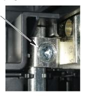
b. Tighten the clamping screw 1/4 turn at a time, <u>verifying for movement after each 1/4 turn</u>, until the connector does not move anymore. When the connector will not move anymore, apply a mark with the black permanent marker, between the connector and clamping screw. See Figure 17.
