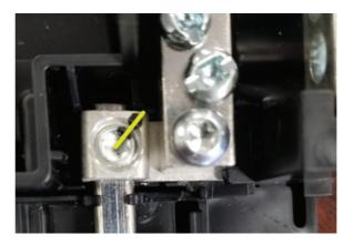
c. <u>USING THE TORQUE WRENCH, RE-TIGHTEN</u> the right bottom neutral bar screw to 25 lb-in. (2.8 N•m). Add mark to the right bottom neutral bar screw with black permanent marker. See Figure 18.
