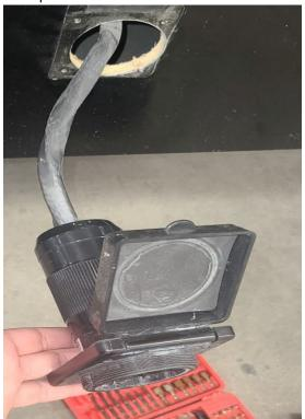
15. Now tighten the screws in the socket until snug (careful not to strip the screw or hole)
