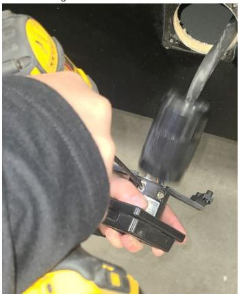
9. Remove inlet from wires
