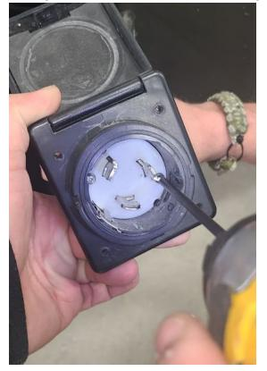
16. Now push the inlet back in to its hole on the coach and install the four #2 square screws and reseal around the inlet if necessary.
