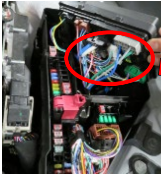
IPDM inside the engine room
