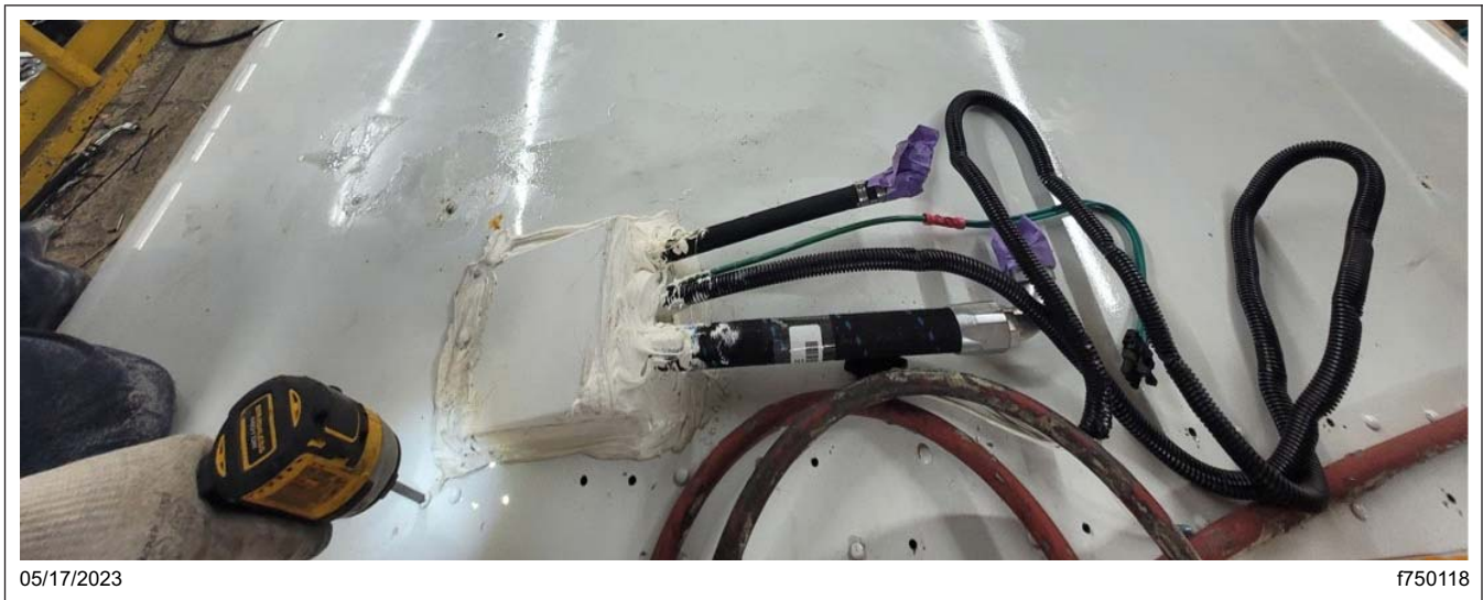
Fig. 14, Installing the Screws along the Joint
