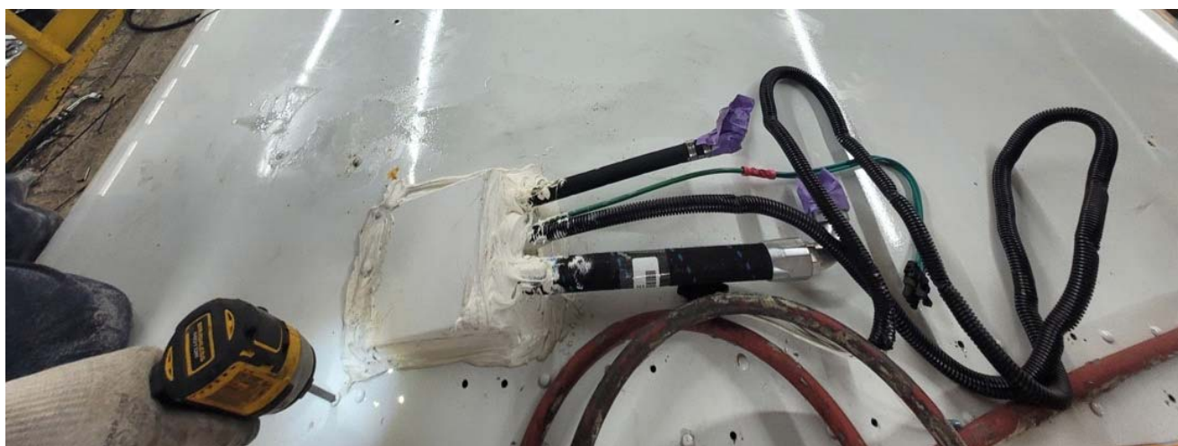
Fig. 14, Installing the Screws along the Joint
