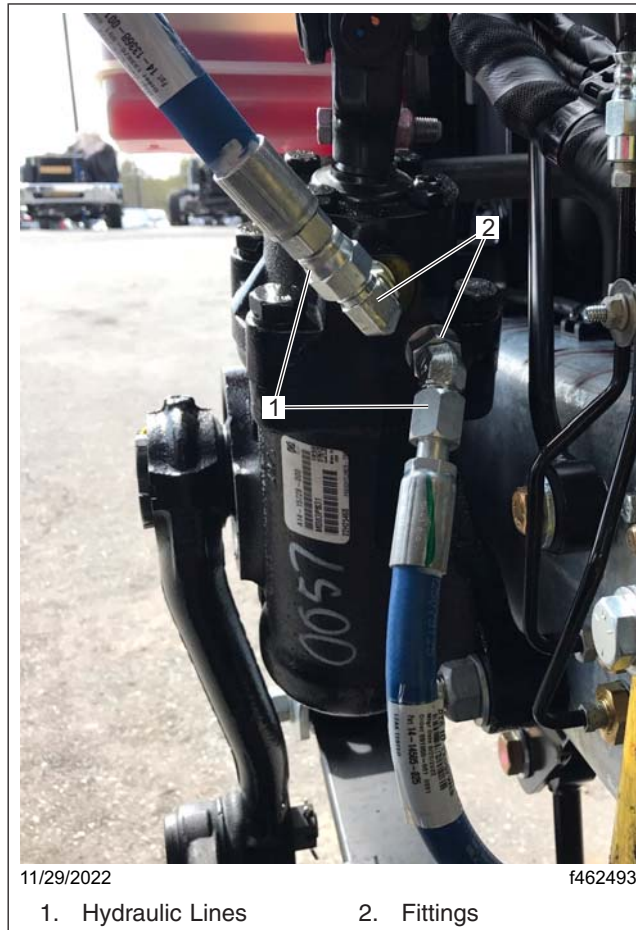
Fig. 8, Hydraulic Lines Removal
