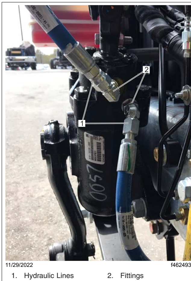
Fig. 8, Hydraulic Lines Removal
