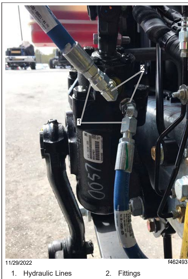
Fig. 8, Hydraulic Lines Removal
