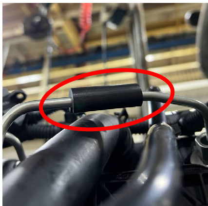
Figure 3: Example of the gap that should be present between the Vibration Isolator on Fuel Injector Supply Line #5 and the Crankcase Breather Tube
