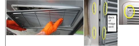
Reinstall vent by lining up the tabs on the right side of the frame with the slots in the grill and pivot the left side in. Push top clip down and install screw into metal plate (be careful not to strip the screw). Push bottom clip down until it locks onto plastic tab (you should hear it "click" into place).
