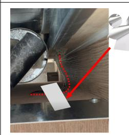
Remove the backing from the foil tape and secure the wire against the outer wall, away from the fridge flue.
