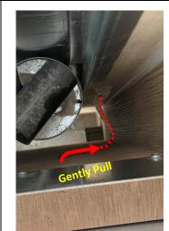
Reach in and with your hand, move the wire away from the exhaust flue by pulling from the outer wall.
