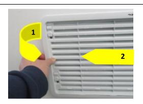
Lift both tabs up and remove vent by pulling on the left side of the vent and then sliding it out. Set vent aside.
