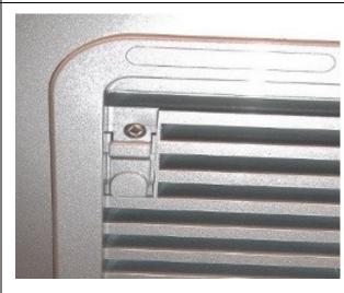
Push both sliding clips down and fasten the vent cover through the original hole with the original screw.
