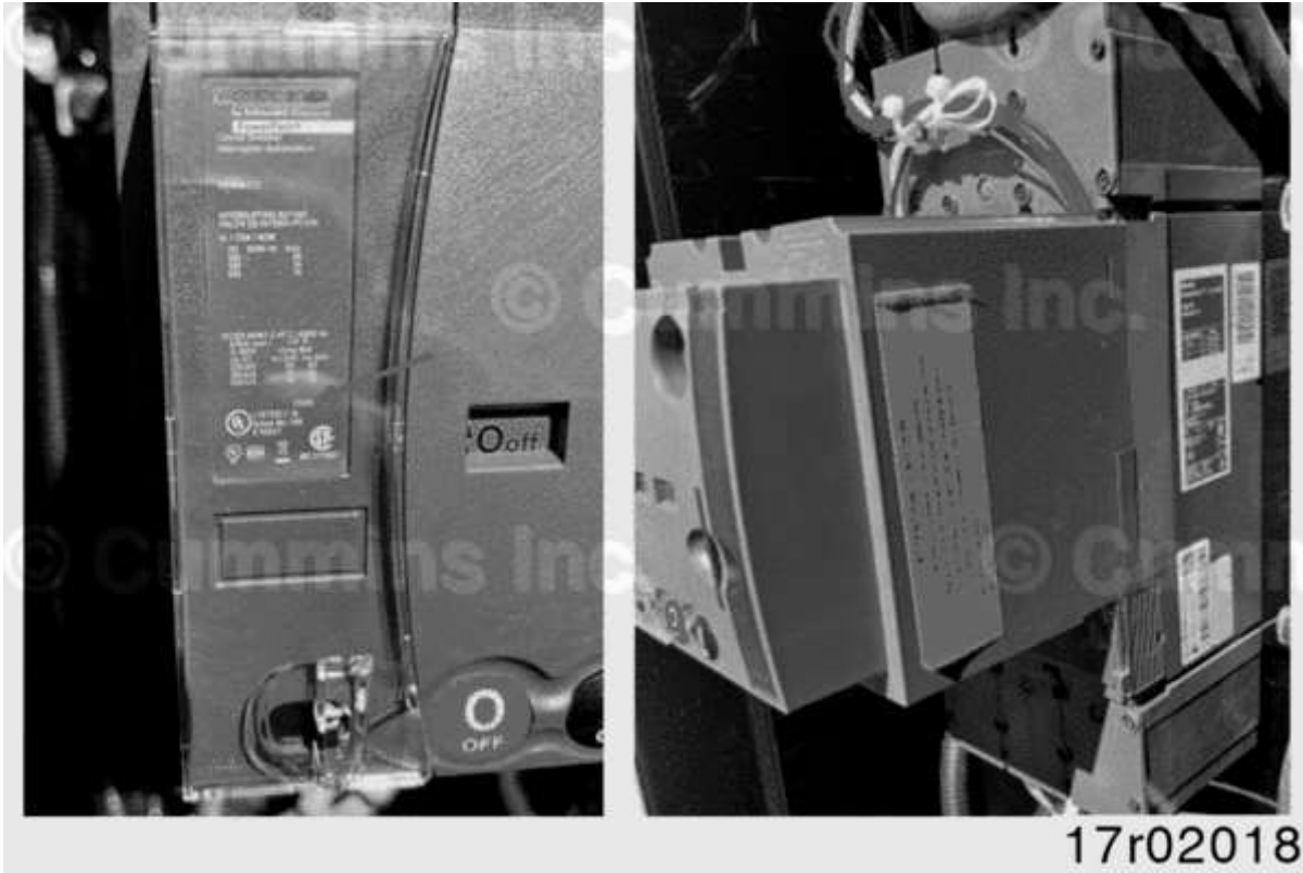
Figure 4, Breaker Date Code Location on A055A272
