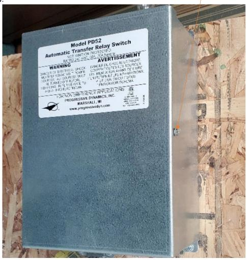
4. Once cover has been removed from the transfer switch using an in.lbs torque screwdriver /wrench tighten each conductor lug to the specified torque indicated on the inside of the transfer switch cover or in the installation instructions.
