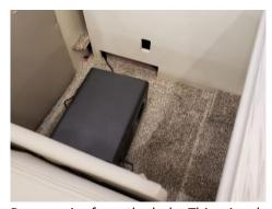
4. Pull the Romex wire from the hole. This wire should be labeled "OUTLET."
