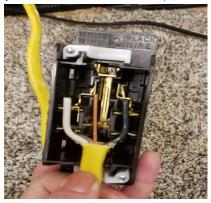
6. After installing the outlet, reinstall the dinette and secure the outlet with 2" screws to the exterior TV cover cabinet. (This can also be mounted in the cabinet itself if an outlet size hole is cutout.)
