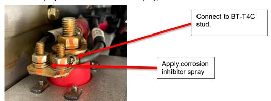
40. Attached reworked equalizer cables to fuse holder BT-125/BT-126. Ensure a smooth curve from the equalizer to the fuse holders. Torque studs to 40 IN-LBS.
