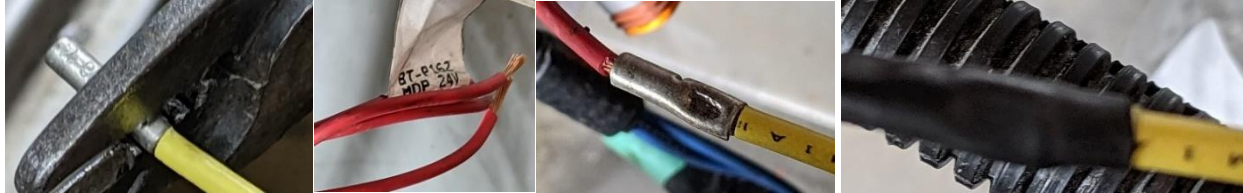
Crimp butt splice
