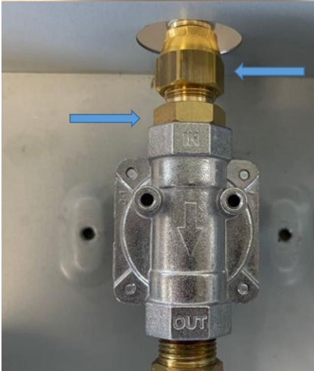
Use a 3/4" and 5/8" wrench to tighten the LP connection.
