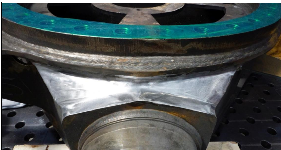
Illustration 09-53- 11: Working area prepared for installation of reinforcing plate
