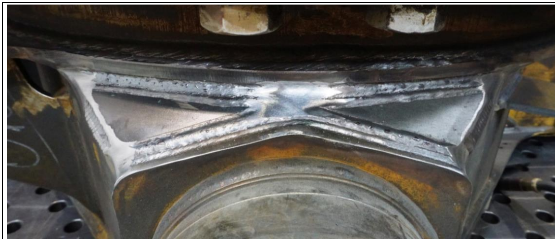
Illustration 09-53- 30: Grinded weld run outs
