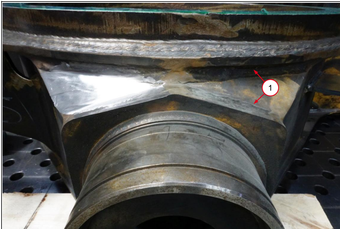
Illustration 09-53- 10: Welding seams ready to install reinforcing plate
