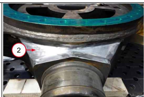
Illustration 09-53- 4: Grinded welding area, ready for repair work
