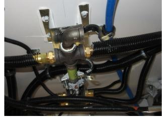
Thread in street elbow to face the direction the hose was routed.
