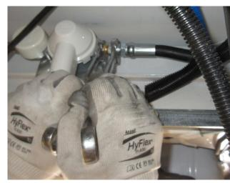
Re-attach the other end of the hose to the regulator with two wrenches.
