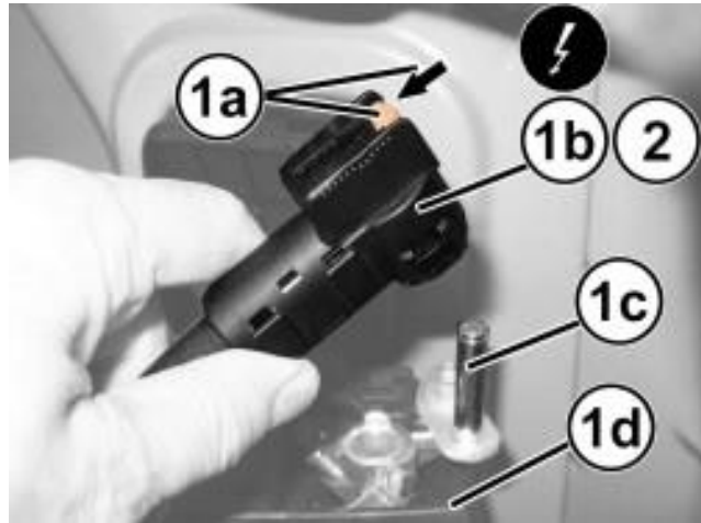
Figure 19 – Battery Negative Cable
