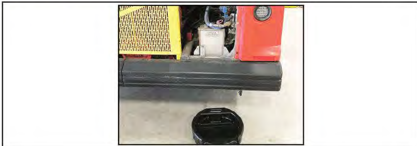
Figure 1 - Place Container to Collect Hydraulic Oil
