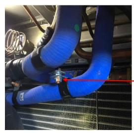
Remove and save bolt, nut and clamp
