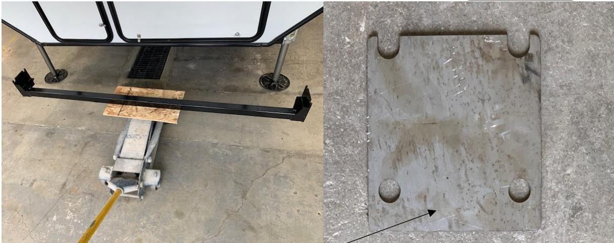
15. Use the provided shims that are 1/8" & 1/4" thick to ensure that the bracket has no more than a 1/2" gap to be closed up when tightening bolts. (Some brackets may not require any shims & will have less than 1/2" gap once in place)
