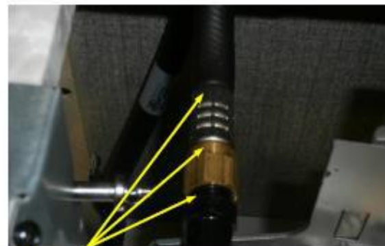
INTERIOR COOKING APPLIANCE; REMOVE TOP OR PULL OUT FROM CABINET OPENING TO HAVE FULL VIEW & ACCESS TO THE CONNECTION ⚠️ LIBERALLY APPLY BUBBLE SOLUTION @ EACH OF ALL 3 AREAS. OBSERVE FOR 30 SECONDS.
