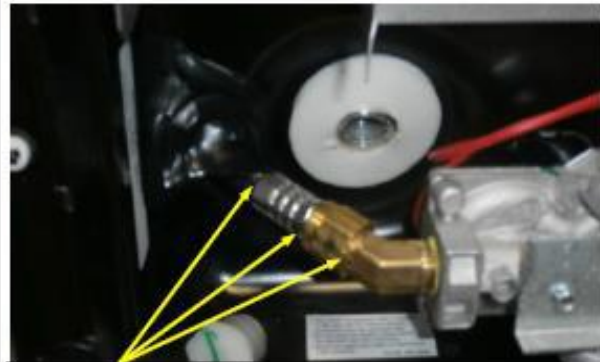
WATER HEATER; ⚠️ LIBERALLY APPLY BUBBLE SOLUTION @ EACH OF ALL 3 AREAS. OBSERVE FOR 30 SECONDS.
