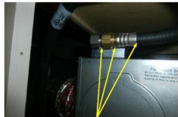
FURNACE; REMOVE RETURN AIR GRILL ⚠️ LIBERALLY APPLY BUBBLE SOLUTION @ EACH OF ALL 3 AREAS. OBSERVE FOR 30 SECONDS.
