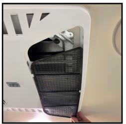
Reinstall the air conditioner shroud using the six (6) screws retained earlier.
