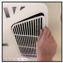
Locate and remove six (6) screws holding the shroud to the air conditioner unit. Retain for later use.
