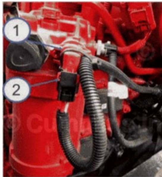
Figure 4: Removing Cable Tie and Disconnecting the Fuel Heater
