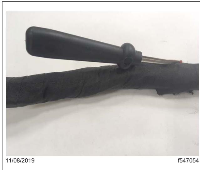
Fig. 4, Cutting an Opening into the Fiber Wrap
