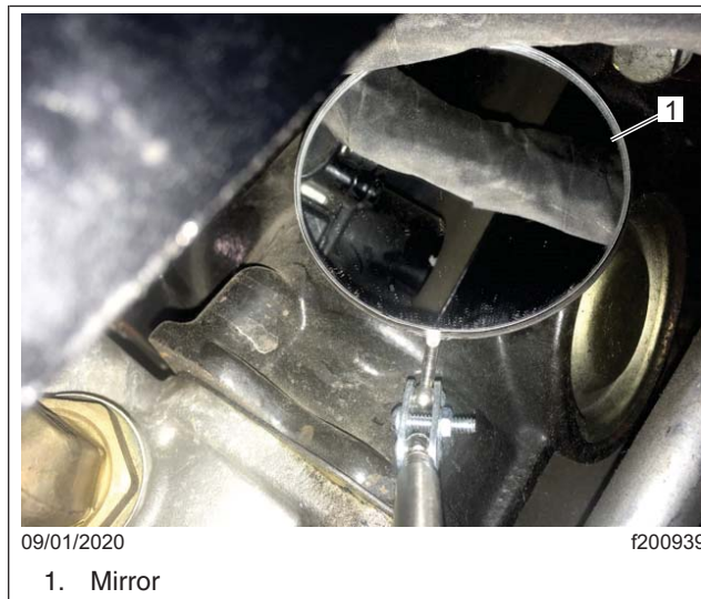
Fig. 3, Inspection by Mirror
