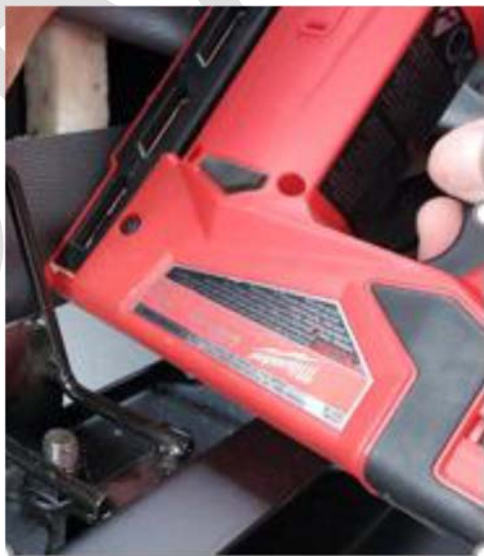
Figure 11: Staple vinyl from back to wooden stick all the way across
