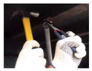
• Finally, inspect the newly attached Zinc and yellow colored beam clip to ensure it is fully attached and the spring is hanging straight.
