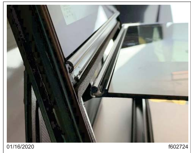
Fig. 2, Window Dropped Out of Hinge
