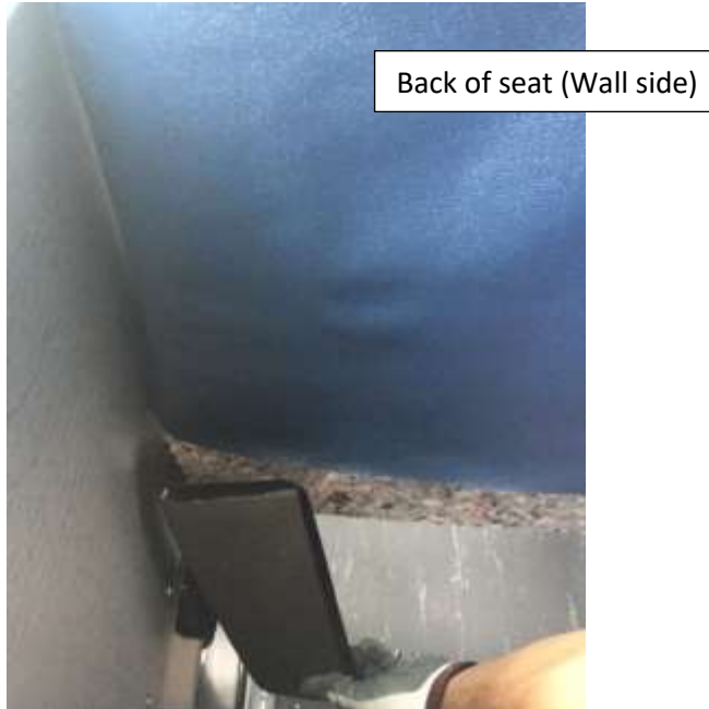
Figure 6: Positioning the Repair part in place
