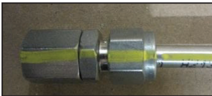
Figure 40: Yellow paint mark on the trigger line components.
