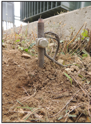
Illustration of a grounding rod in the ground.
