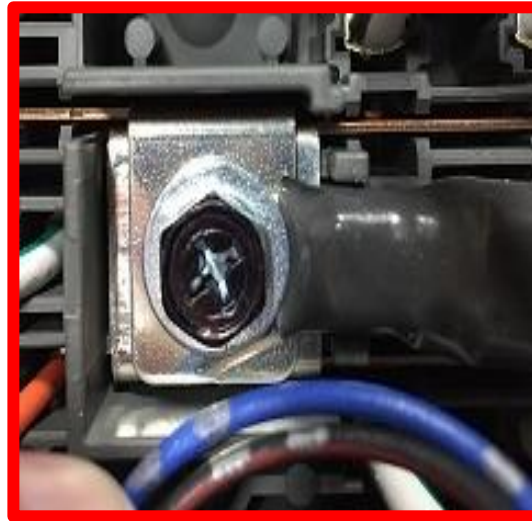
Figure 11 – Not OK Condition
