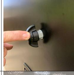
From the interior side, place one large washer and one large nut on the latch mechanism and tighten to the exterior skin. This can be done using the 1 1/16" deep well socket.
