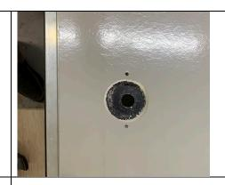
From the door exterior, use the 7/8" hole saw to cut through the exterior skin.
