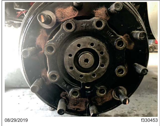
Fig. 7, Removed Flange Bolts that connect the Drive Flange to the Wheel Hub
