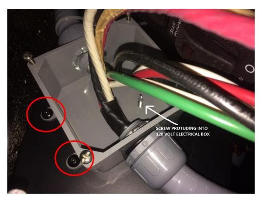
6. Caulk the hole in the junction box that was left from removing the screw to prevent any water intrusion.
