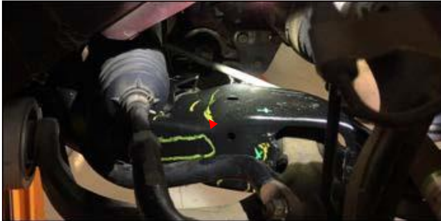
Top Side View: Non-Damaged Cross Member
