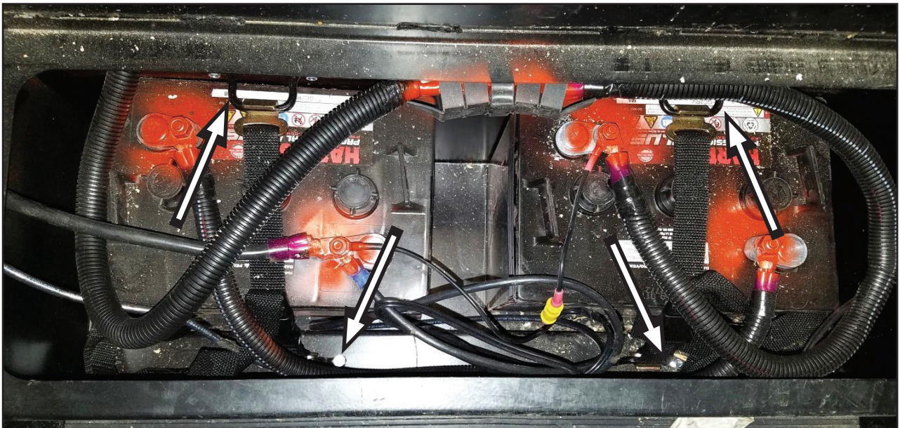
Figure 5 Arrows indicate original locations of the (4) battery hold down strap mounting brackets
