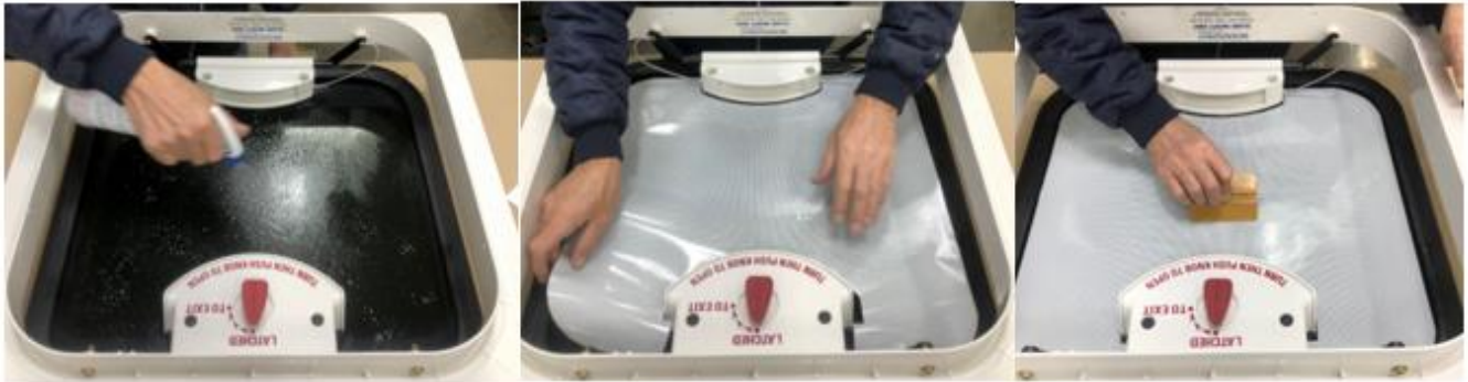
Figure 4: Apply a soap and water solution to the interior surface of the glass and place the tint film.
