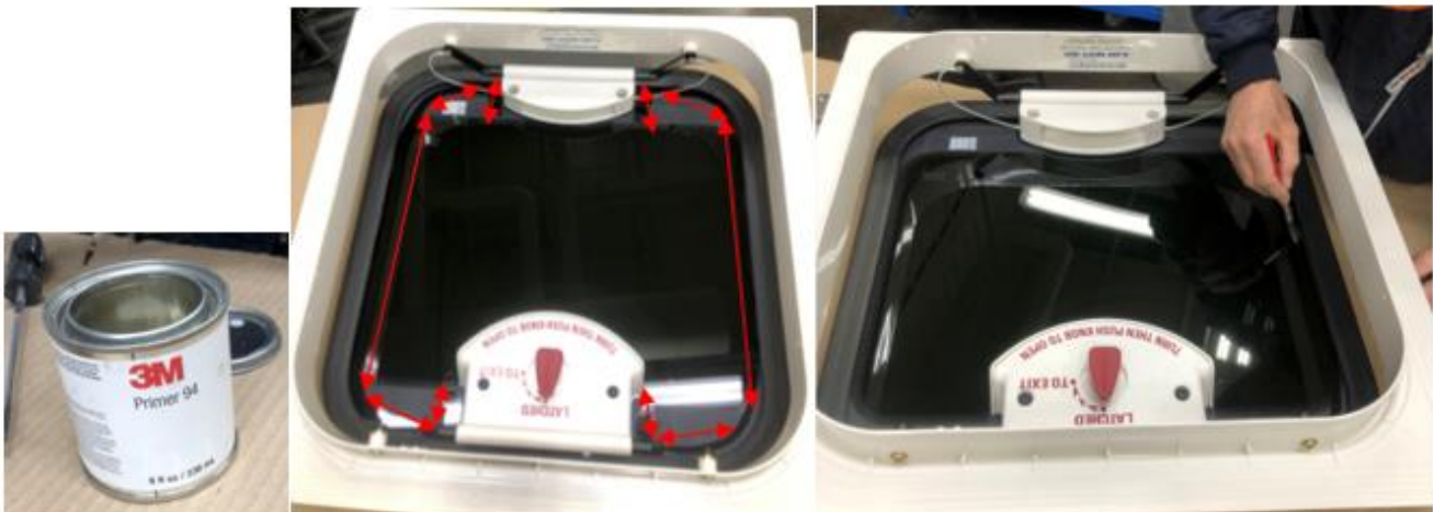
Figure 3: Apply #94 Primer - PN 356274 on the interior side of the glass panel, as denoted by the arrows.
