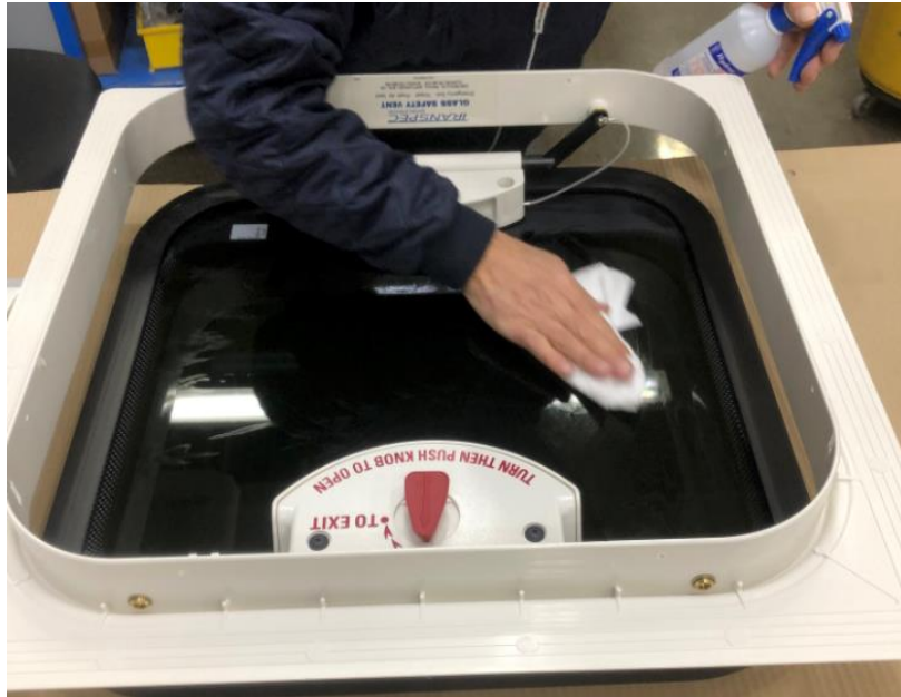
Figure 2: Clean the interior surface of the glass with a clean, lint-free cloth and isopropyl alcohol.
