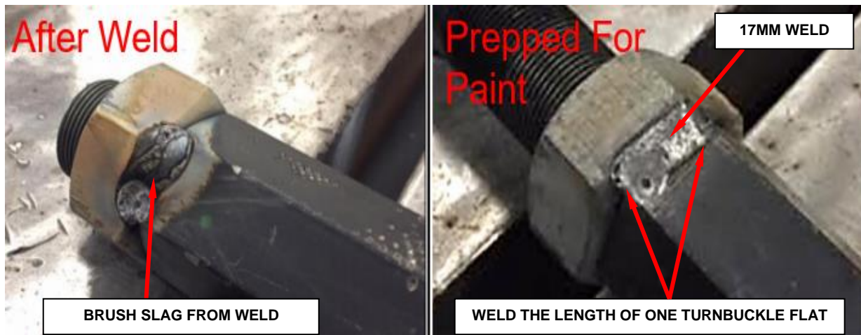
Figure 10 – Prepare areas for Paint
