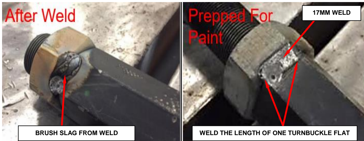
Figure 10 – Prepare areas for Paint
