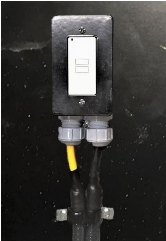
Figure 17. AFCI/GFCI device installed under bunk
