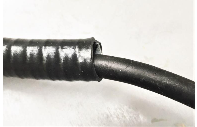
Figure 7. Conduit trimmed to length and free of sharp edges
